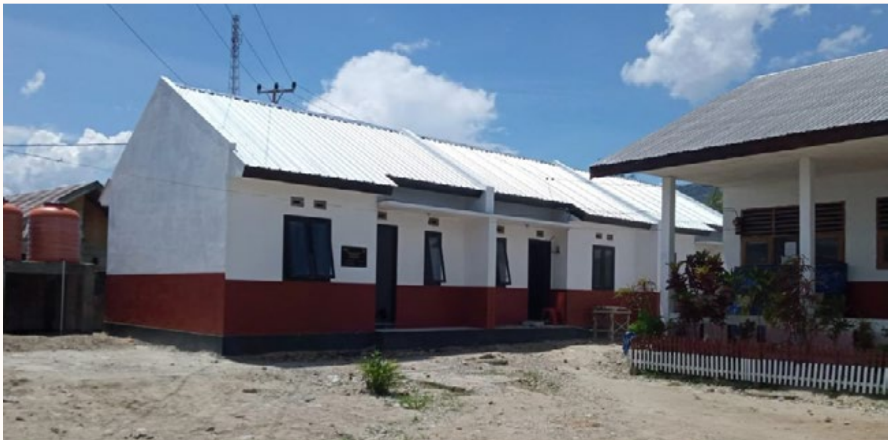
THE REFURBISHED SCHOOL IN LAWUA VILLAGE
